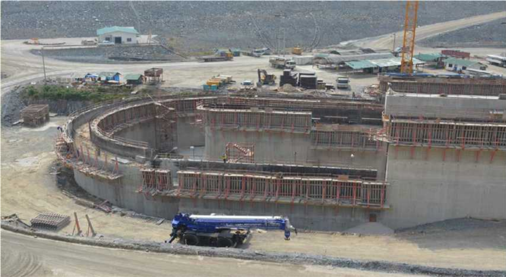
Ongoing concrete work at the fish ladder early 2016
